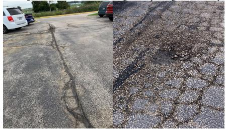
Add drainage for bus parking area. This is the area where we had a bus tire that had ice that froze around the tire. Water floods the area between the light pole and the storage shed flowing onto the asphalt and pooling in the bus tire indentations created from the weight of the bus in the summer when the asphalt
